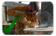
Use appropriate tools and personal protective equipment (full-face mask, safety boots, gloves, overalls) when welding.
