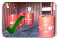
Disused fuel tanks awaiting recycling should be stored at a safe distance from potentially flammable materials and spark sources and over a protected hard surface.
