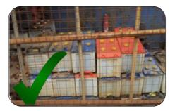
Drain used batteries and store them in a well-ventilated and enclosed area, on a hard surface. Avoid stacking more than three lines of batteries, and no more than 50 batteries in the same location at a time.
