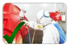
Use the appropriate personal protective equipment (PVC gloves, safety boots, protective overalls) with a hood and an air -purifying respirator.
