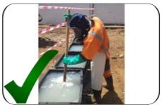
Acid must be drained, neutralized with baking soda and put in a sealed, plastic container. Neutralized acid should be transported to a hazardous waste facility. Metal and plastic parts can be recycled through an authorized contractor.
